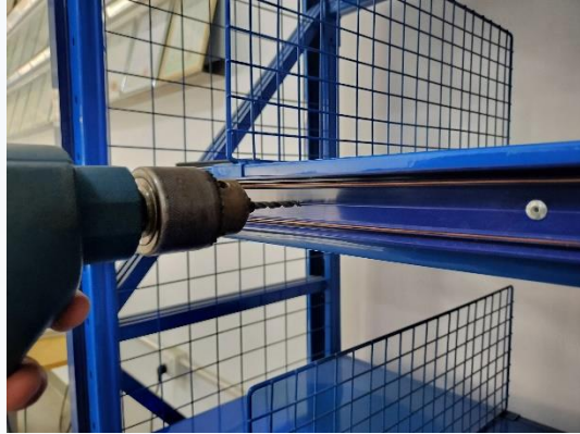
1、 Drill holes on the rack to install duct
